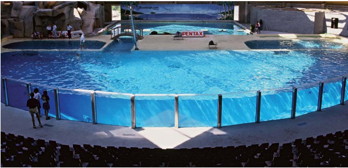
These steel dry-side mullions provide structural support for the silicone butt-joint panels in this exhibition pool. To protect the silicone sealant on the wet-side of the panels from the dolphins, each mullion clamps over the top of the panel with a protective covering inside the pool.
