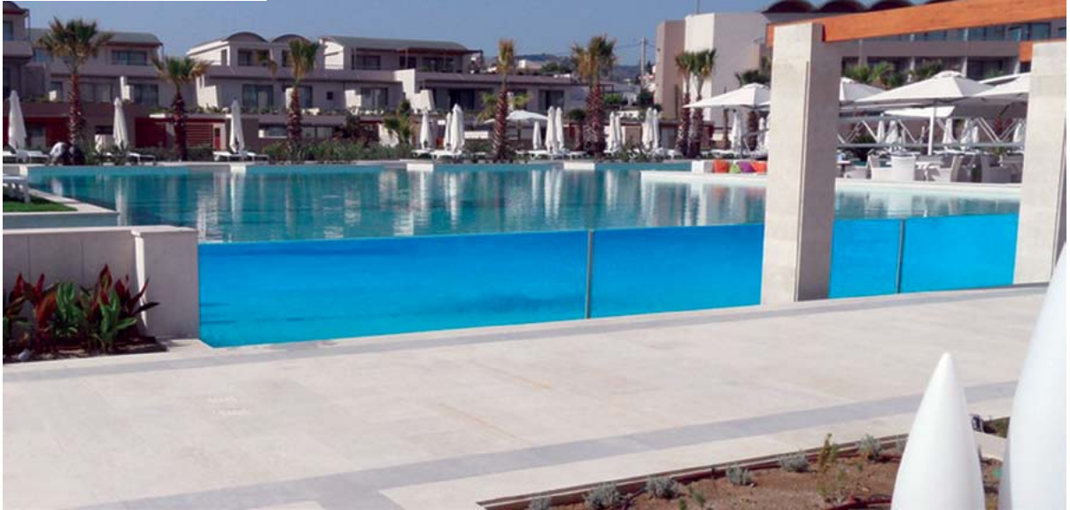
The sealant joints between the panels in this pool allow for larger views directly into the water while using multiple smaller panels. The sealant minimizes the amount of obstructed views while maximizing overall window size.
